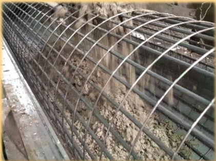
投料 (PURING CONCRETE)
